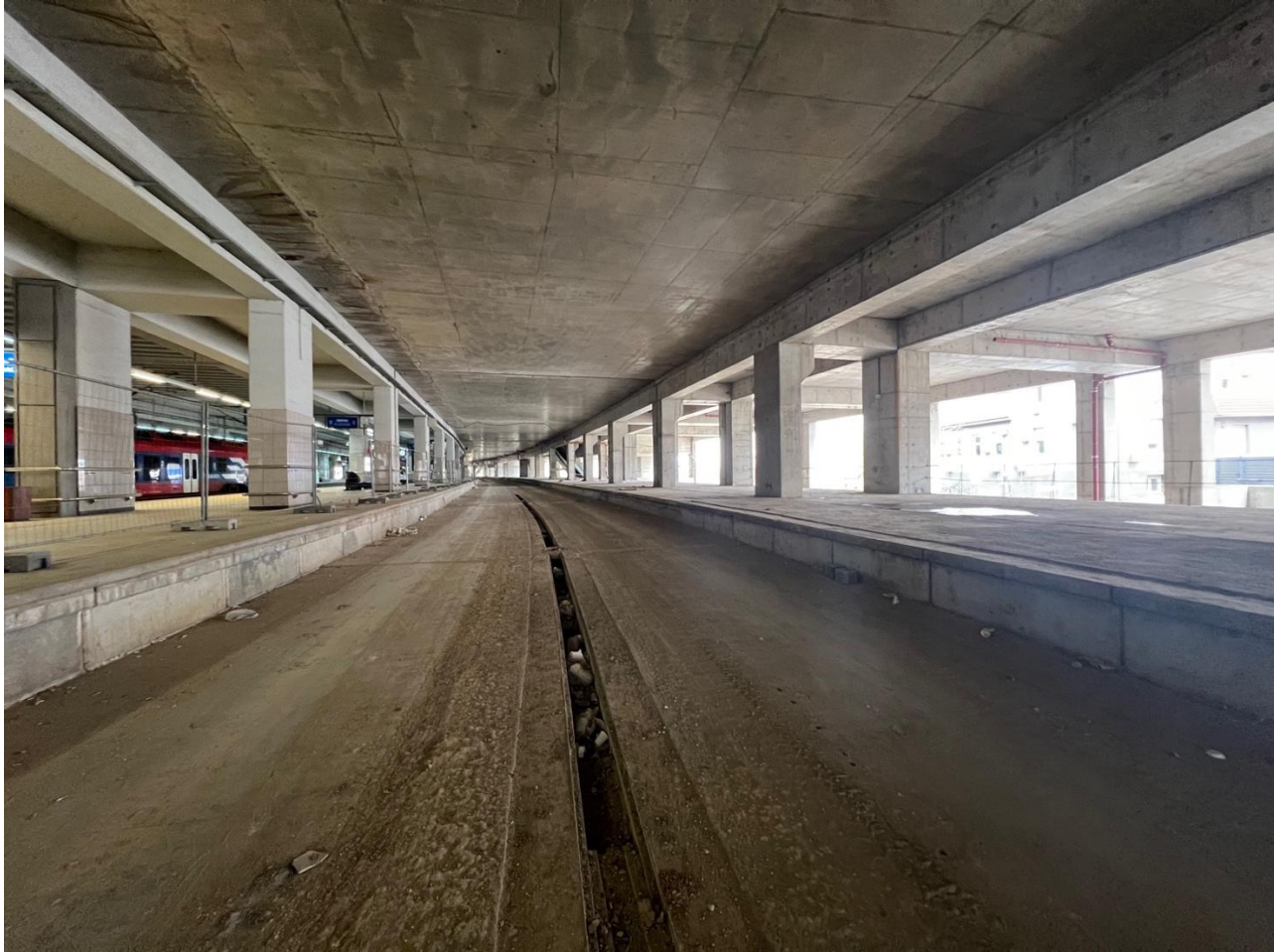
Figure 4: Below the Prokop station ground floor - platform on which finishing works will be carried out and railway tracks where new rails will be placed as part of the SRSM subcomponent project
